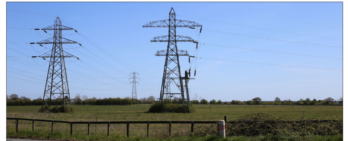
Multiple overhead lines are present in the view to the south-west of the viewpoint.
